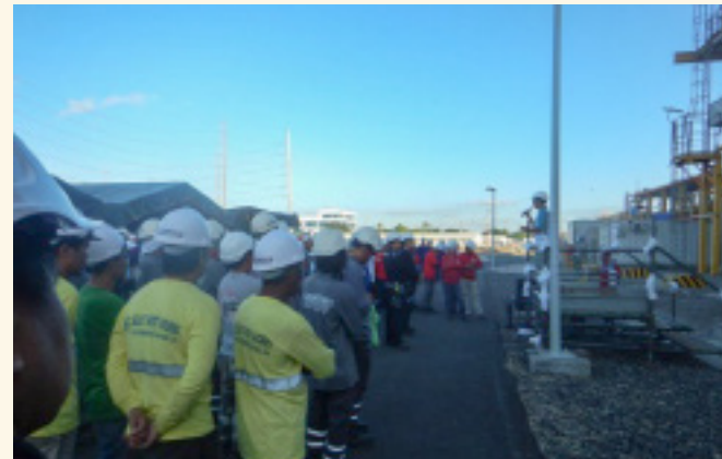
Early morning Toolbox Talks include a safety orientation and reminders for the workers to use personal protective equipment
